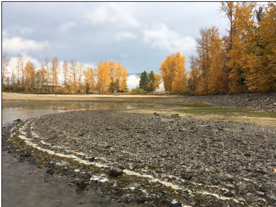
Figure 4. Low water survey condition at 10BR1026; view north-northwest from near BNSF bridge approach.
