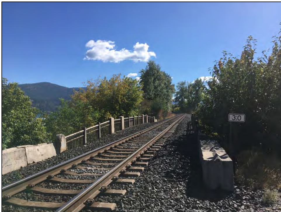
Figure 29. BNSF Bridge 3.1 Railing; View South
