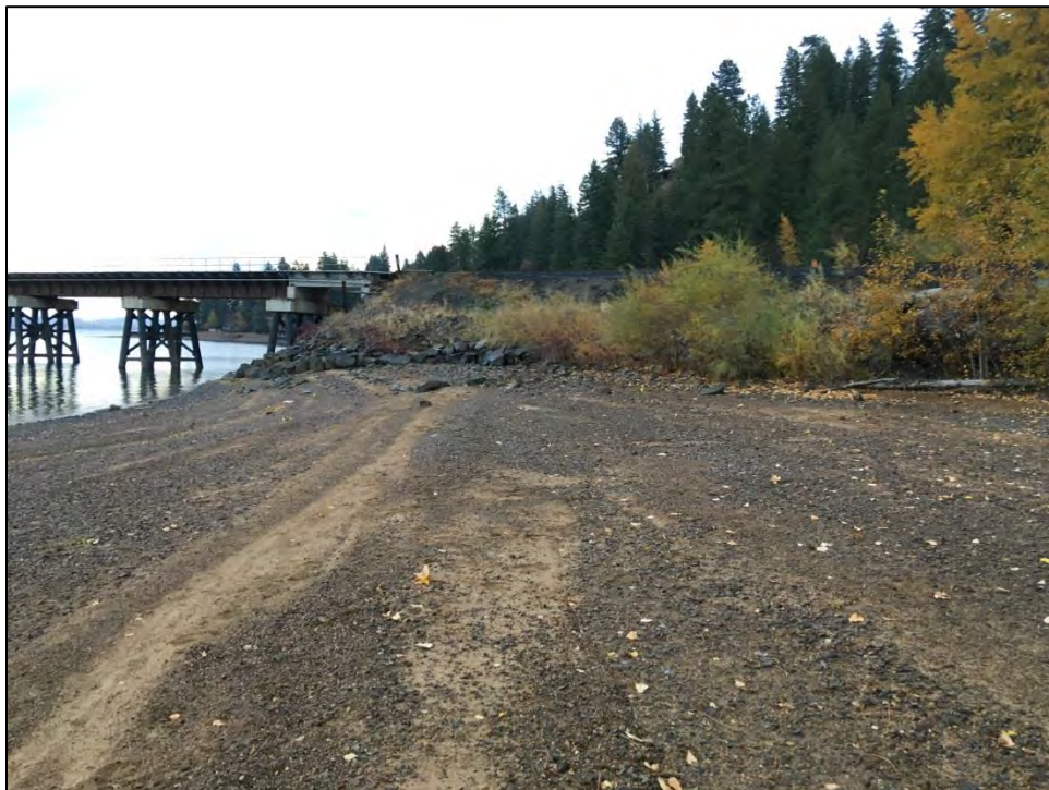
Figure 20. Survey Surface Conditions below OHWM at Bridge 3.9 South End
