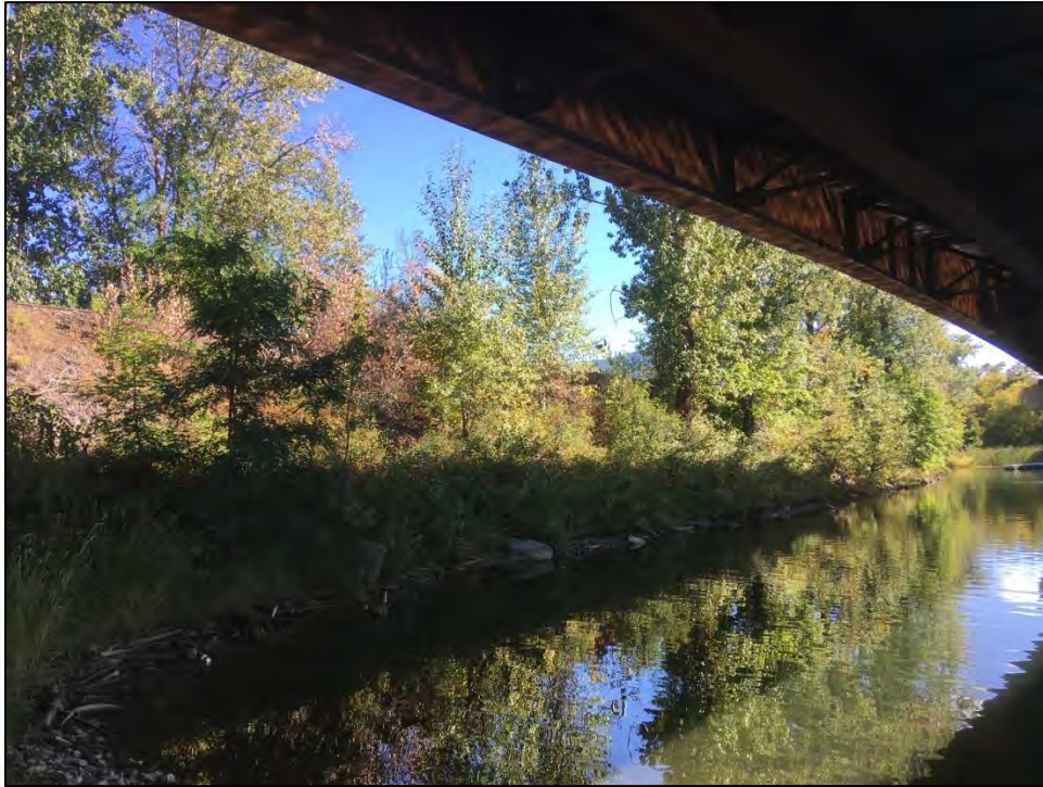
Figure 11. Railroad Fill Prism South of Bridge 3.1; Bridge Overhead is US 95; View to Southeast
