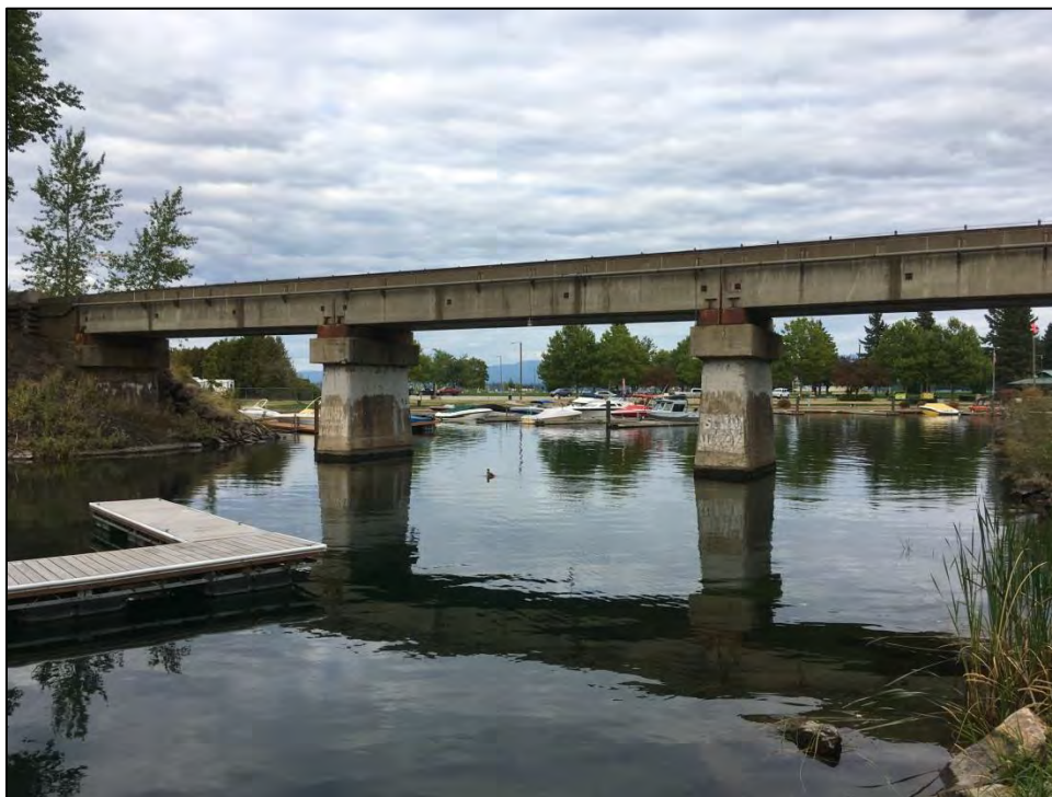
Figure 32. BNSF Bridge 3.1, West Elevation
