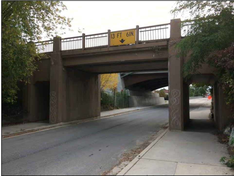
Figure 28. BNSF Bridge 3.0 West Elevation
