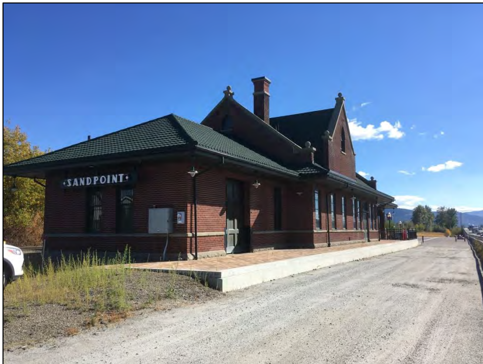
Figure 27. Northern Pacific Depot, North and West Elevations
