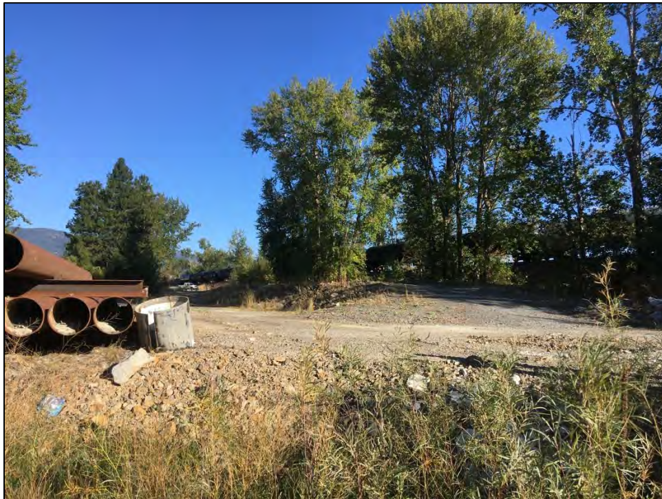
Figure 14. New Fill Immediately North of Dog Beach; View North from Shoreline
