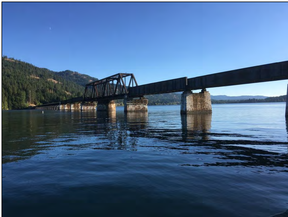
Figure 31. BNSF Bridge 3.9, East Elevation, South Half
