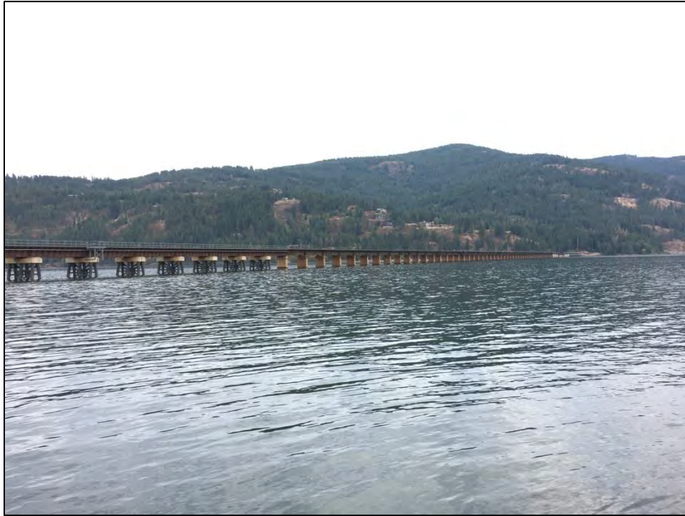
Figure 30. BNSF Bridge 3.9, West Elevation
